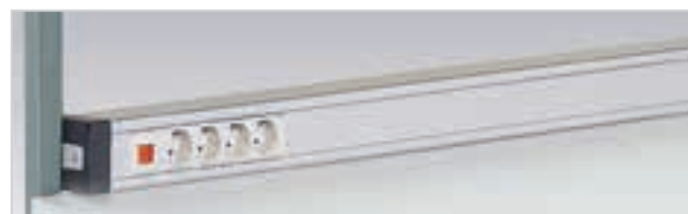
Power channel TJK
